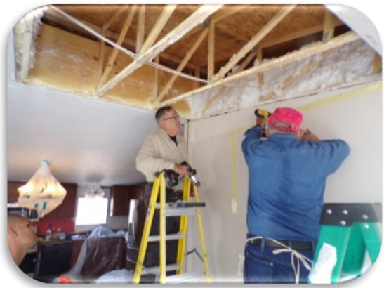
Pete Gomez and Chon Pena helping a Marine in need repair fire damage in his home.
